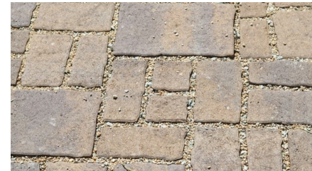
Concrete pavers with gaps for infiltration
