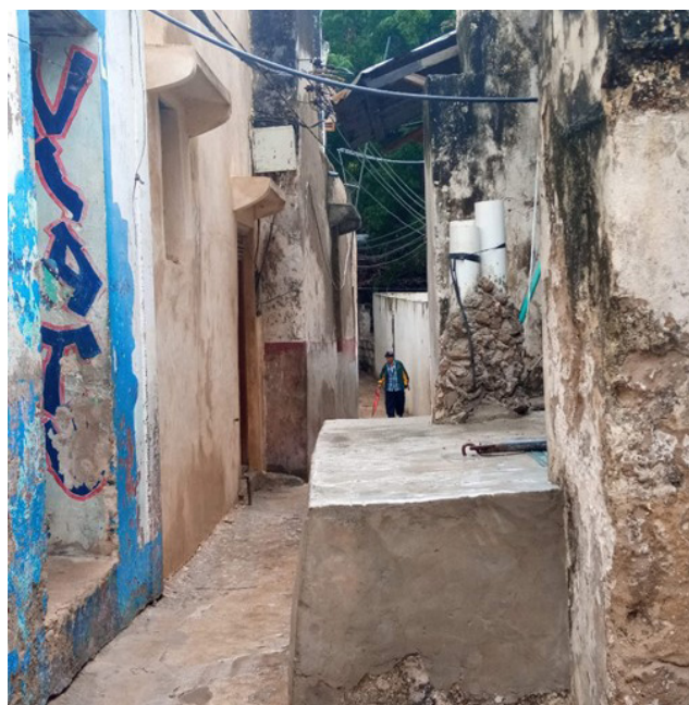
Figure 4.47 Domestic septic tank constructed on the street
