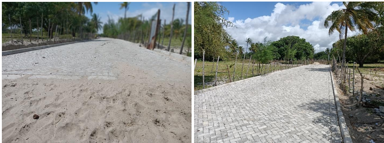
Plate 3-8: Cabro road under construction through the NCDF and KeRRA to connect Lamu and Matondoni settlements
