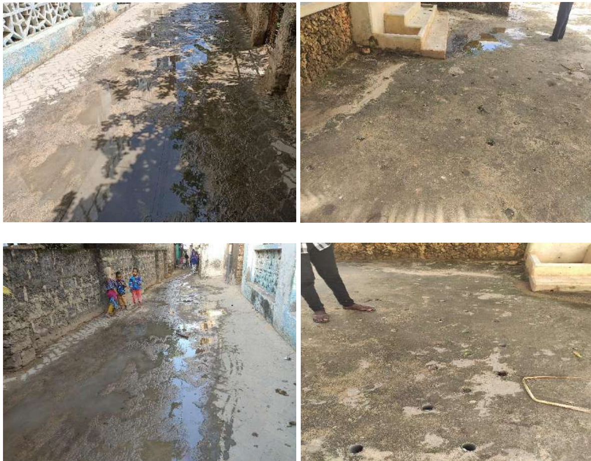
Plate 3-10: Shows Timamy road in Shella which is poorly drained and, on the right, some of the soak pits
