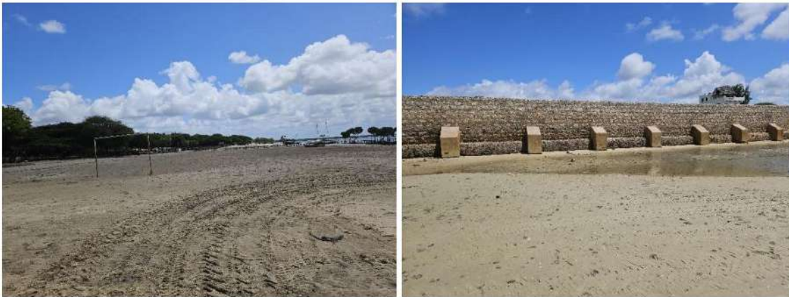
Plate 5-3: Public Sporting Area; Retaining Wall in Wiyoni's Seafront
