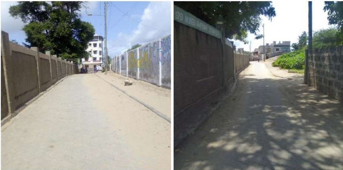
Plate 4-10: Cabro-paved Streets that allow for Motorized Transport within the Outer Buffer Zone
