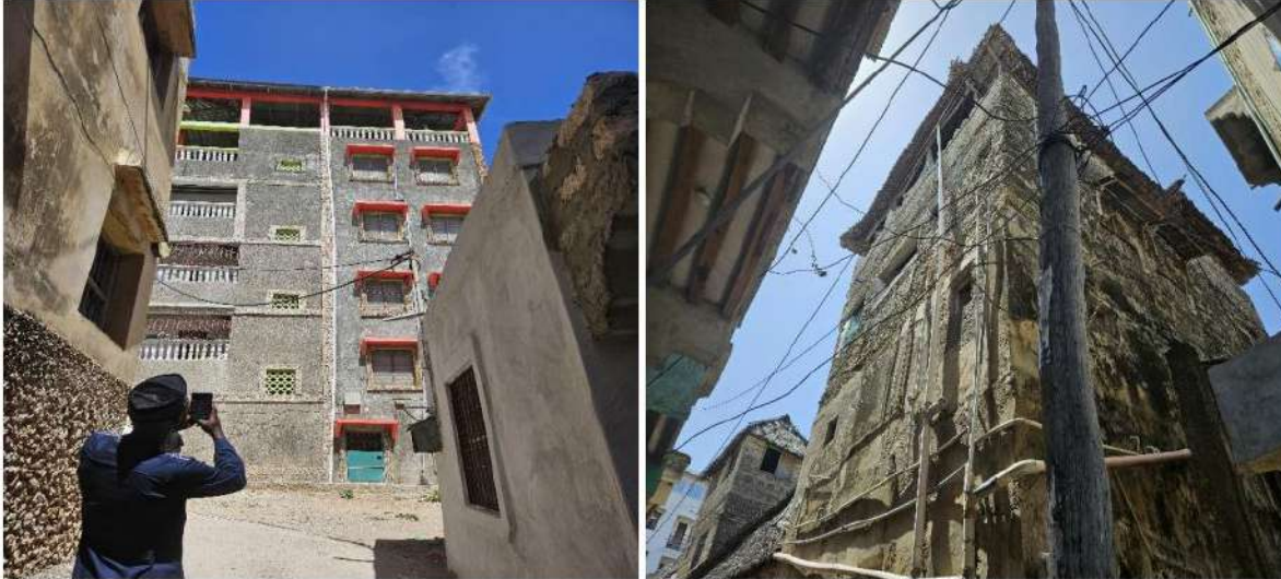
Plate 4-12: A Modern High-Rise Building with Uncoordinated Color Codes; Unregulated Building Works Source: KREIS, 2023
