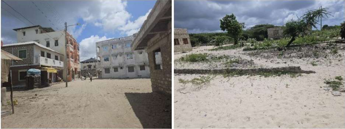
Plate 5-4: Uncoordinated Building Character; Incomplete Building Structures
